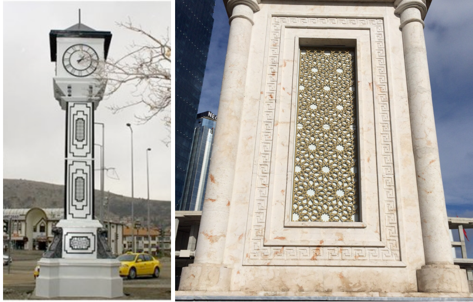
Figure 6 – (Left) Clock Tower in Beypazari, Source: Sak, G. (2014). Beypazari ilçesi de çakma saat kulesine kavuştul!. Türkiye Ekonomi Politikaları Araştırma Vakfı.; (Right) Detail of a Clock Tower near AKP Headquarters showing the use of 12-Point Star Patterns in the Ornamentation, Source: Photo taken by the author
